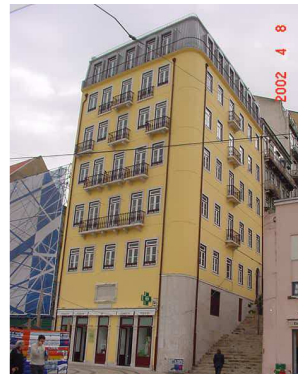
Picture 4 - Rua da Mouraria 8-16 after rehabilitation
