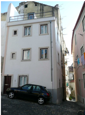
Picture 2 - Largo da Achada, 2 after rehabilitation
